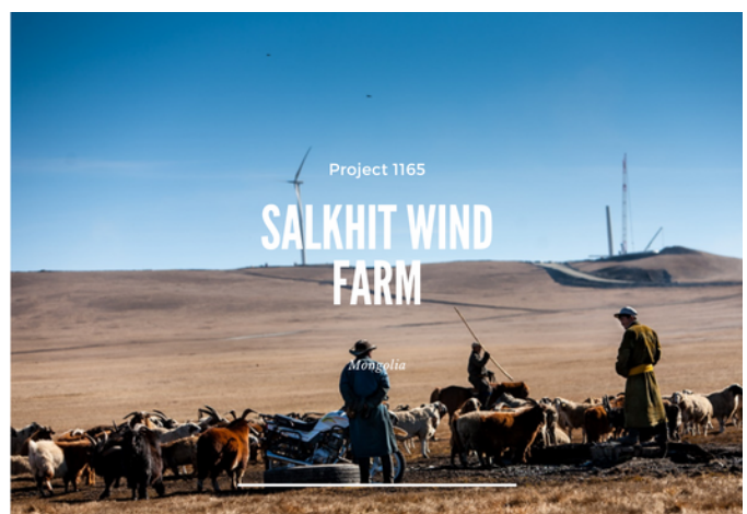
Project 1165: Salkhit Wind Farm in Mongolia
