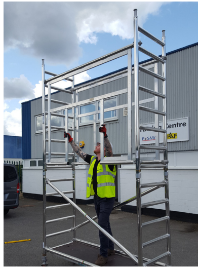
8. Standing on the platform, with the label facing you, position the 1st pair of AGR frames to the uprights with the top hook above the 2nd rung down.
