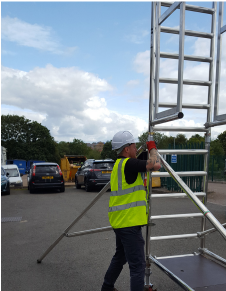
9. Fit stabilisers as early as possible.
