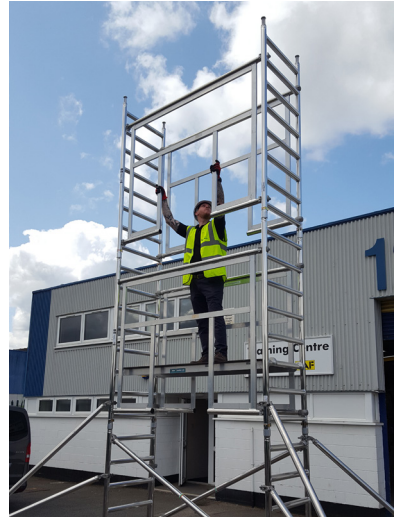
12. Standing on the platform, with the label facing you, position the 1st pair of AGR frames to the uprights with the top hook above the 2nd rung down.
