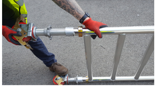
2. Then insert 2 adjustable legs and castor wheels into each base frame
