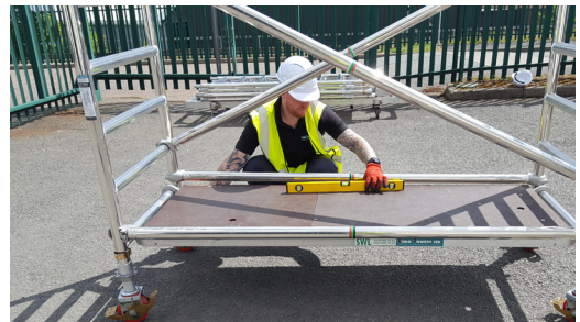
6. Fit a temporary board if required, and then level your tower.
