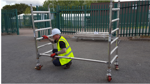
3. Klik in 2 horizontal braces to the vertical member of the frames, as low as possible, above the 1st rung.
