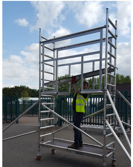
10. Position the trapdoor platform to the rung, 6 rungs down from the top of the frame.
